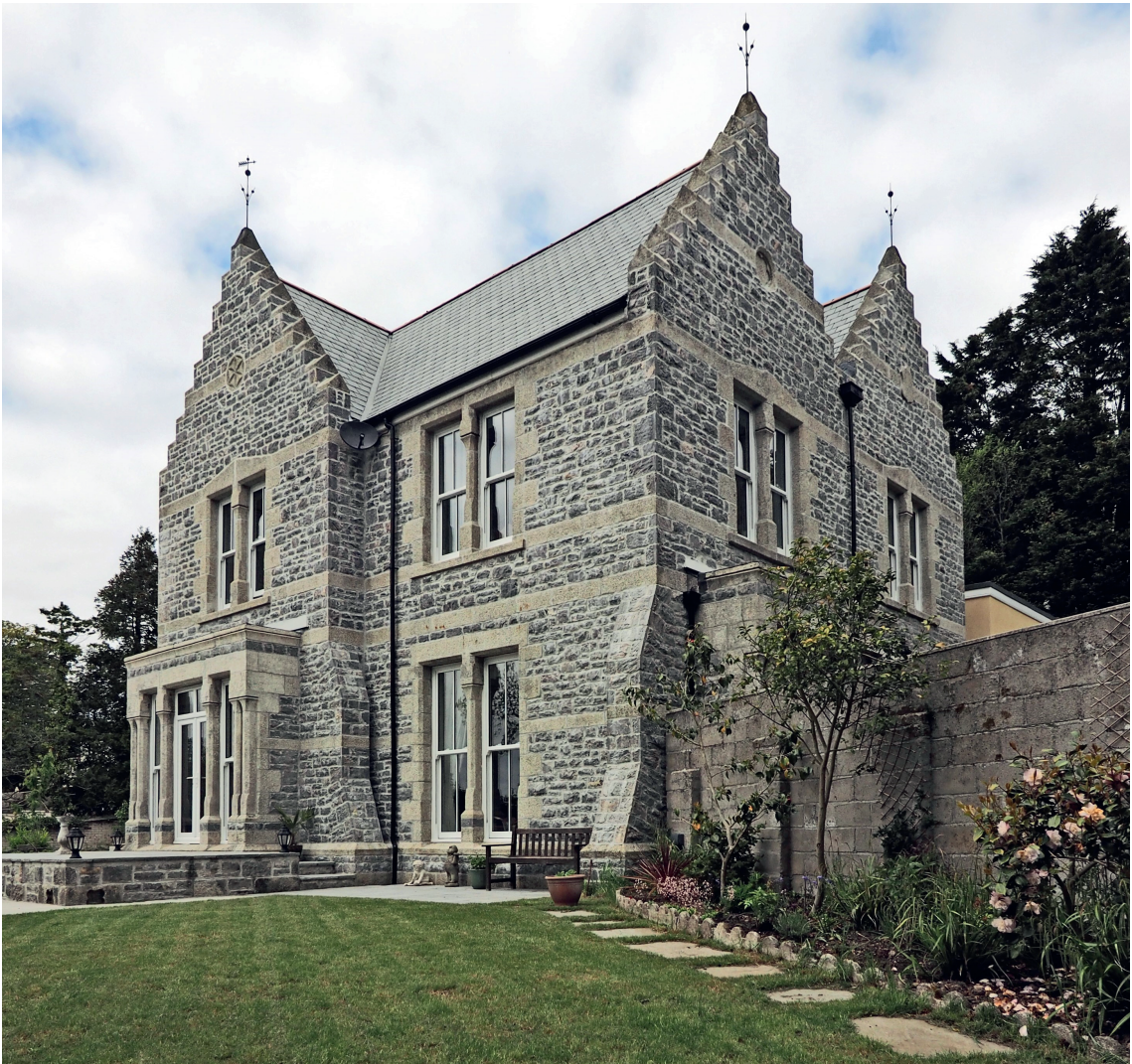
Fig 3 6 Palace Road, St Austell in 2015. Formerly known as Oak Villa and Oakleigh , the house was almost certainly designed by Joseph Ivimey. He was recorded living there in 1867. (Photograph: Eric Berry.)
