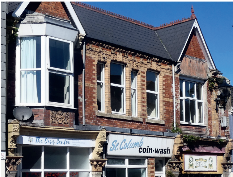
Fig 7 Ornamental detailing in yellow terracotta on the front elevation of 26–28 Fore Street, St Columb Major. Could this be another design by Ivimey? (Photograph: Graeme Kirkham.)
