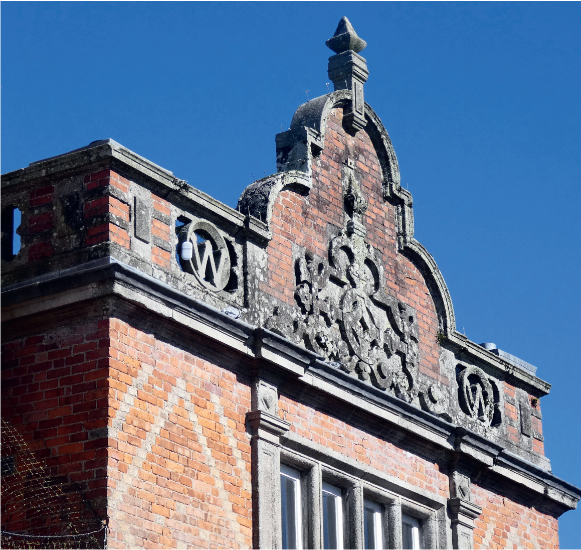
Fig 5 The Dutch-style gable, moulded and pierced parapet and ornamental strapwork on the Broad Street elevation of the bank. (Photograph: Graeme Kirkham.)
