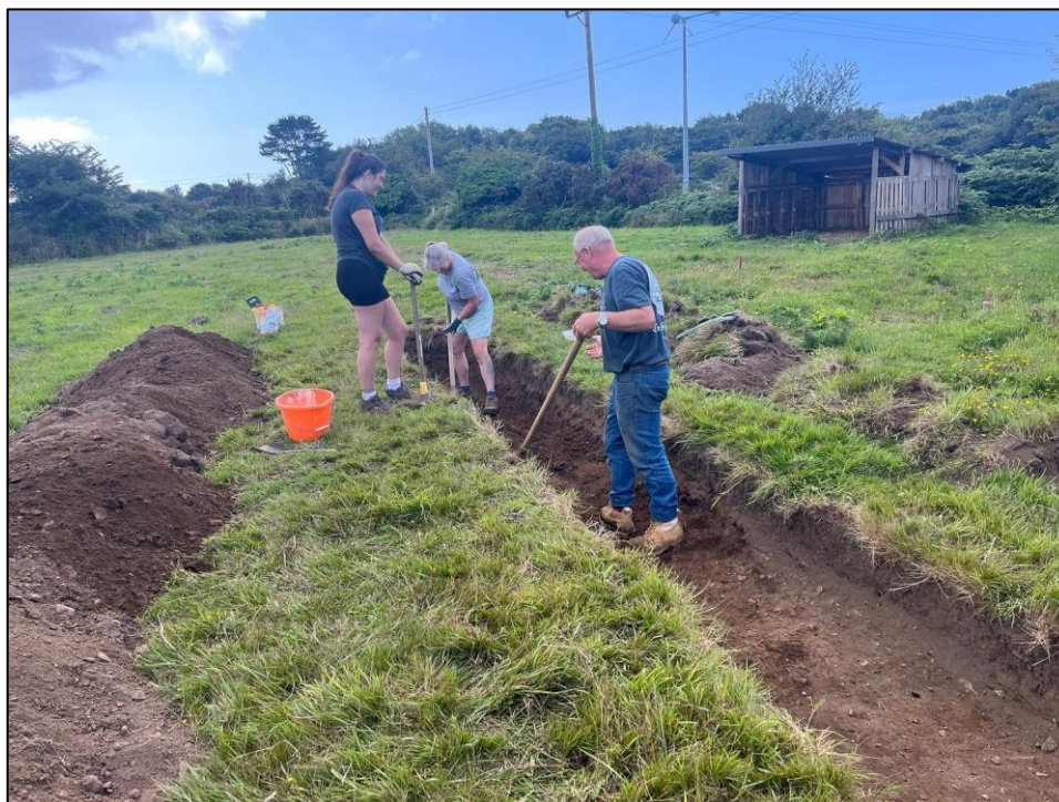
Figure 7: Early days excavating Trench 1.
