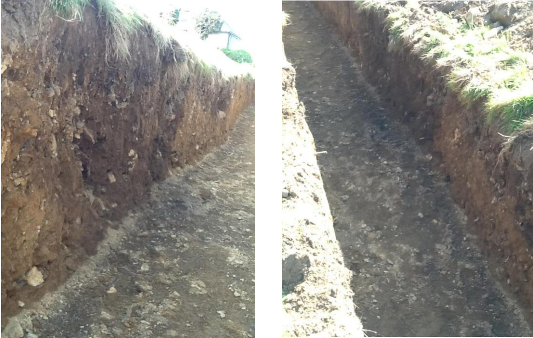
Fig 2 Two views of the potential ditch in the trench excavated by Steve Polglase.
