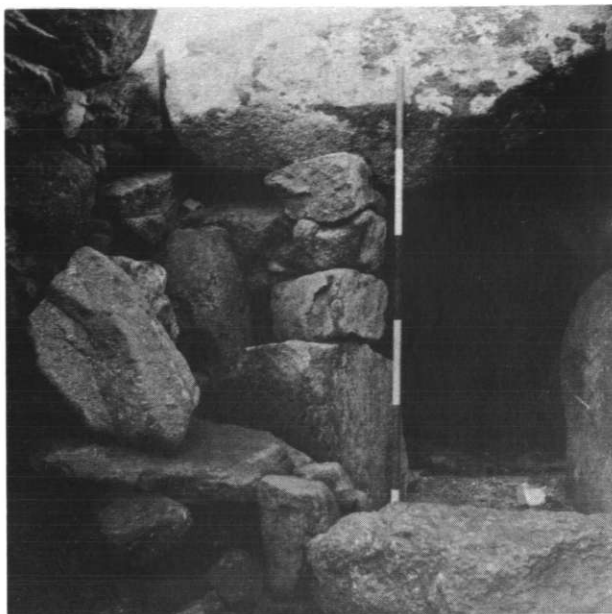
III Fogou: Tipped capstone, supported on pier of stones—seen from East entrance
