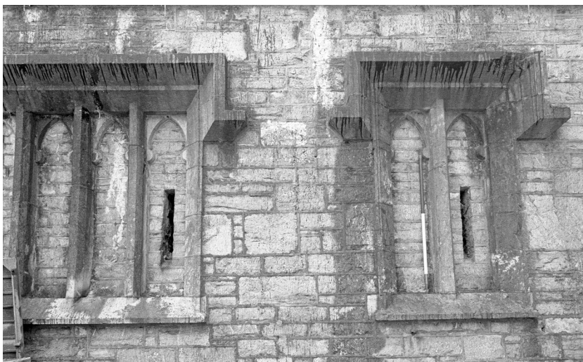
Fig 10 Partially blind windows in the north wall of the men's barracks, showing vents from G5. Scale 1m. (Photographs: Gary Young.)
