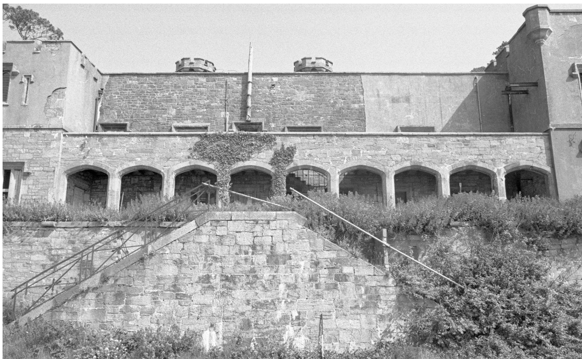
Fig 17 Lower terrace showing steps to upper terrace. Scale 1m. (Photograph: Gary Young.)
