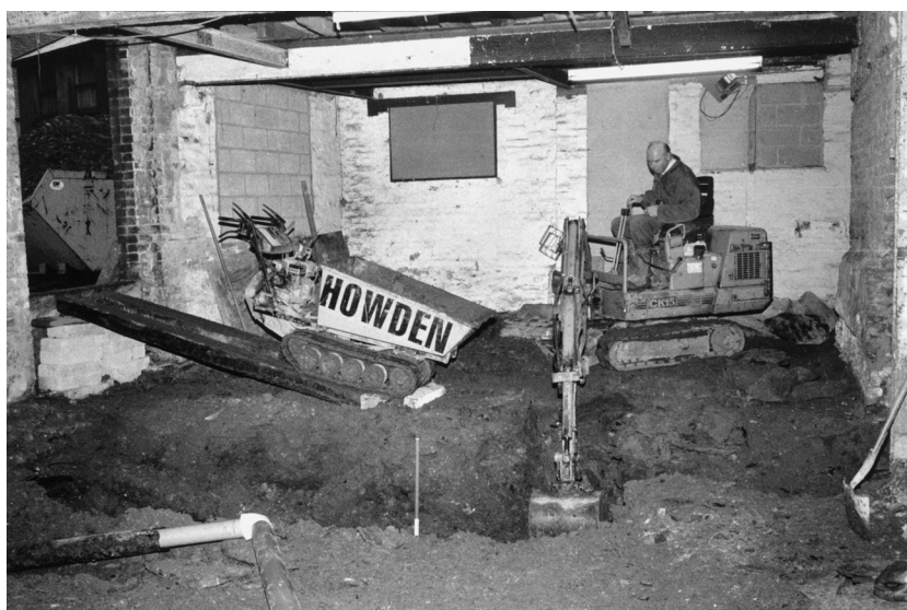
Fig 2 Interior of the building during groundworks. (Photograph: Exeter Archaeology.)
