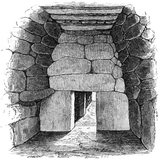
Fig 10 J T Blight's depiction of the northern end of the straight passage, showing the inserted doorway of the extended creep, the doorway at the southern end of the original creep beyond, and the exit to the ditch beyond that (Blight 1885, pl 4). Blight shows the further end of the passage open, at the point where it exits into the enclosure ditch, although it is clear from his description of the site, written in the 1860s, that the ditch was at that time infilled and this access blocked.
