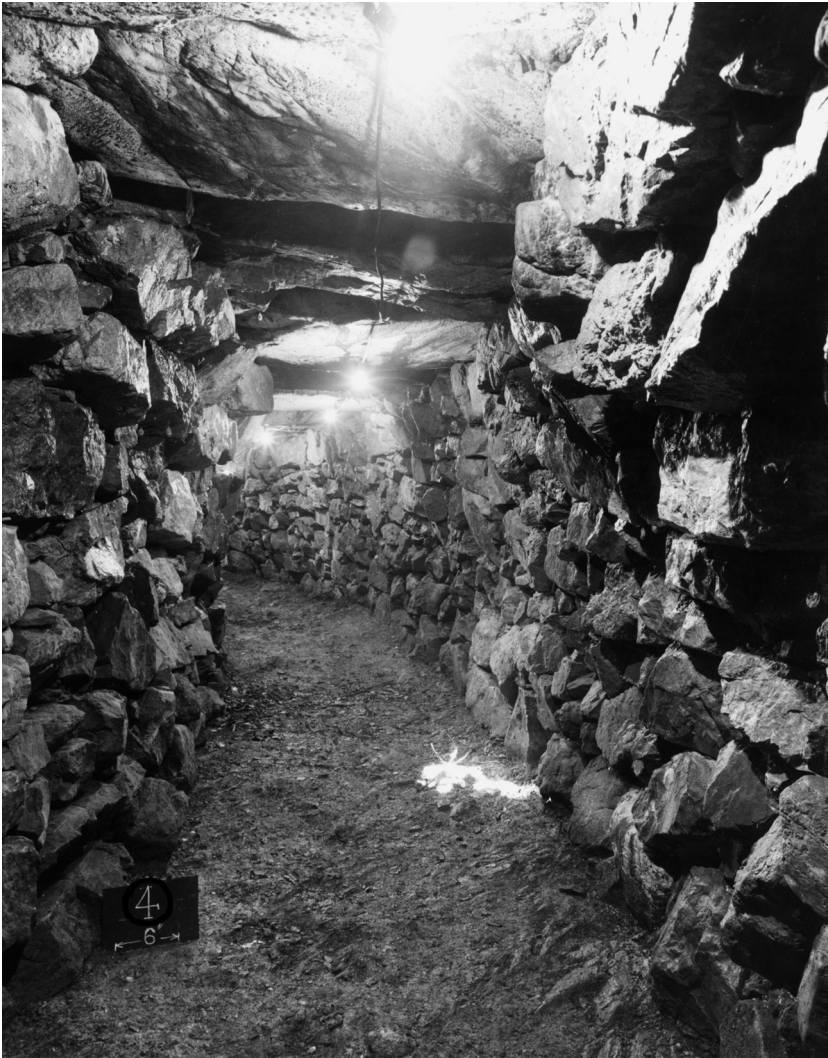
Fig 5 The curved passage, looking south west. (Photograph: Department of the Environment Photographic Section, J95-4-82; 24 March 1982. © Copyright English Heritage.)
