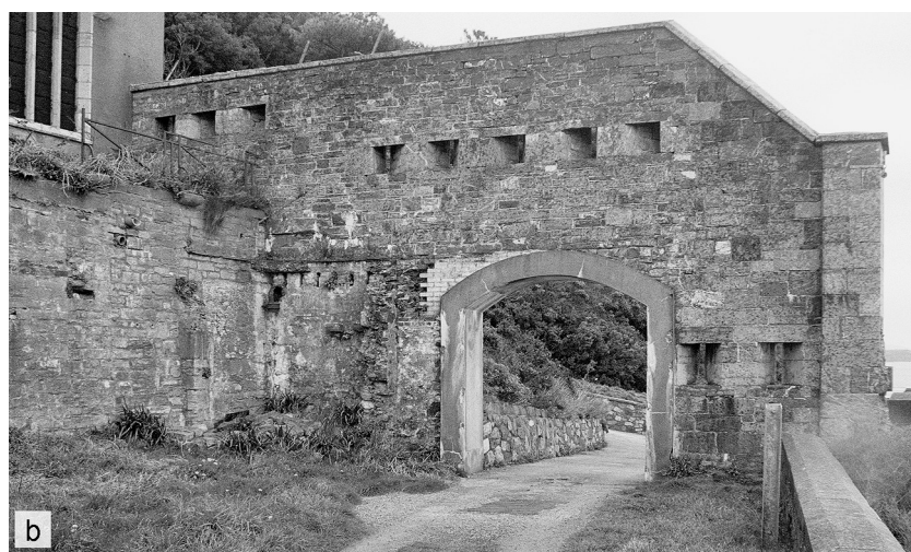
Fig 18 The flanking walls: (a) west (rebuilt), showing entrance to gun battery; (b) east, showing inserted concrete archway. (Photographs: Gary Young.)
