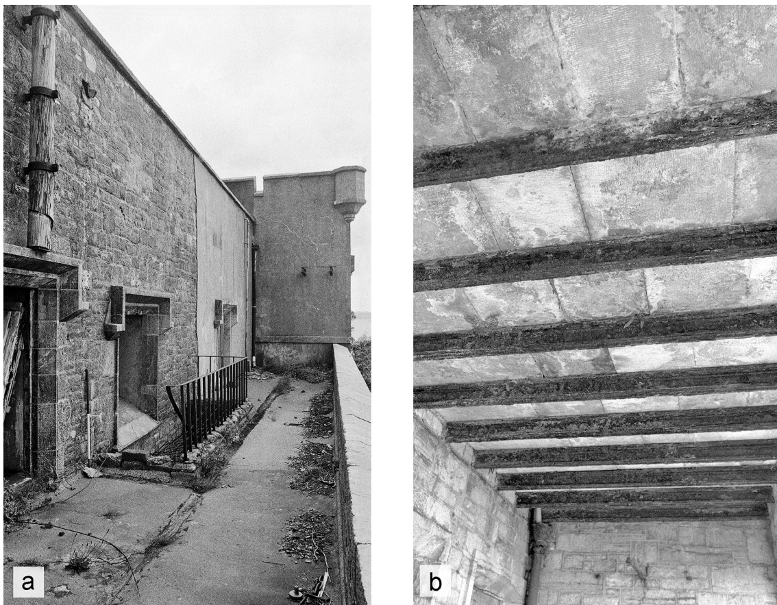
Fig 15 The balcony: (a) stair rising from ground floor, with openings in south elevation of main range and a guérite on corner of east wing; (b) underside showing stone flags supported on cast-iron girders. Scale 1m. (Photographs: Gary Young.)
