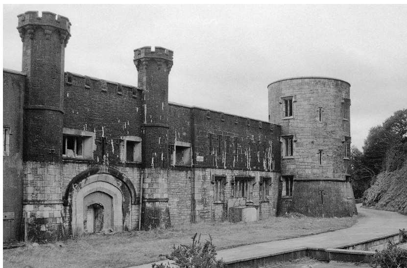
Fig 5 The north elevation, (above) looking south east, (below) looking south west. (Photographs: Gary Young.)
