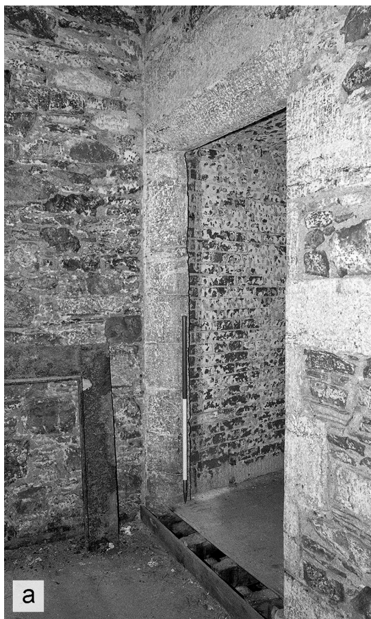
Fig 12 The officers' quarters: (a) entrance from G11 into G15 showing chamfered door jambs and change to brick-lined walls on entry to the officers' quarters; (b) site of stairs in G15 showing panelling. Scales 1m. (Photographs: Gary Young.)
