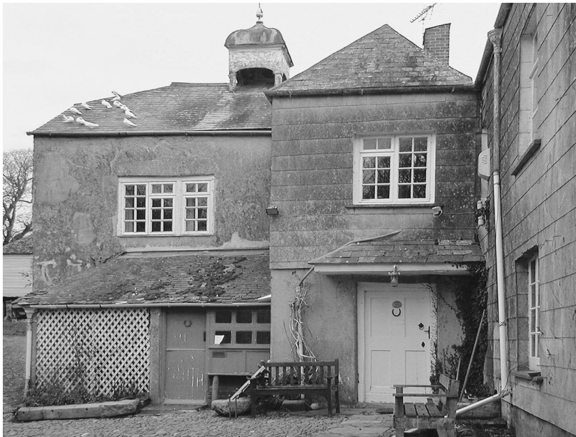
Fig 11 The west range, porch tower and pump house.
