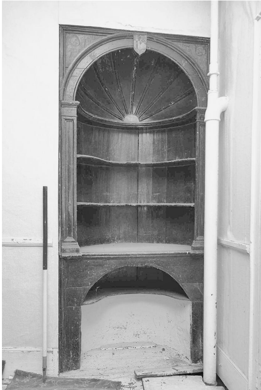
Fig 10 An eighteenth-century cupboard with painted cherubs and heraldic shield in the southern first-floor room of the central range.
