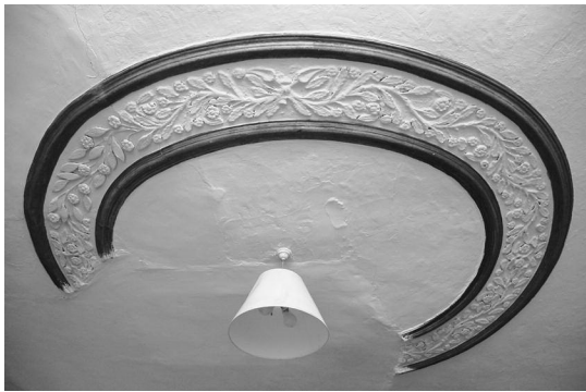
Fig 7 Late seventeenth-century floral plaster wreath in the north room of the central range.
