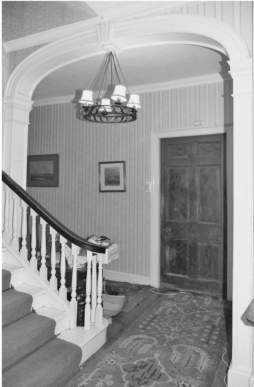
Fig 16 The early nineteenth-century arch in the stair hall of the east range.
