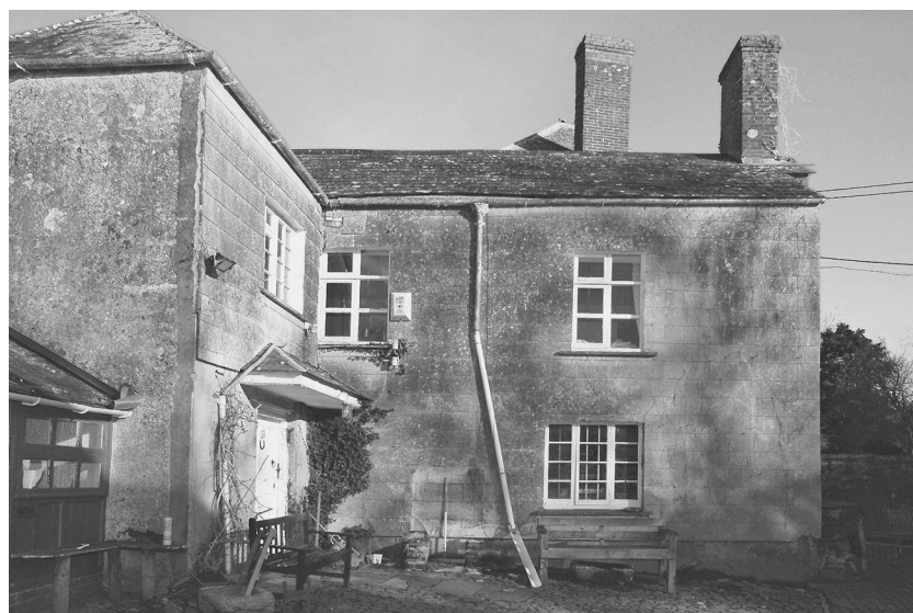
Fig 5 The south-west elevation of the central range.
