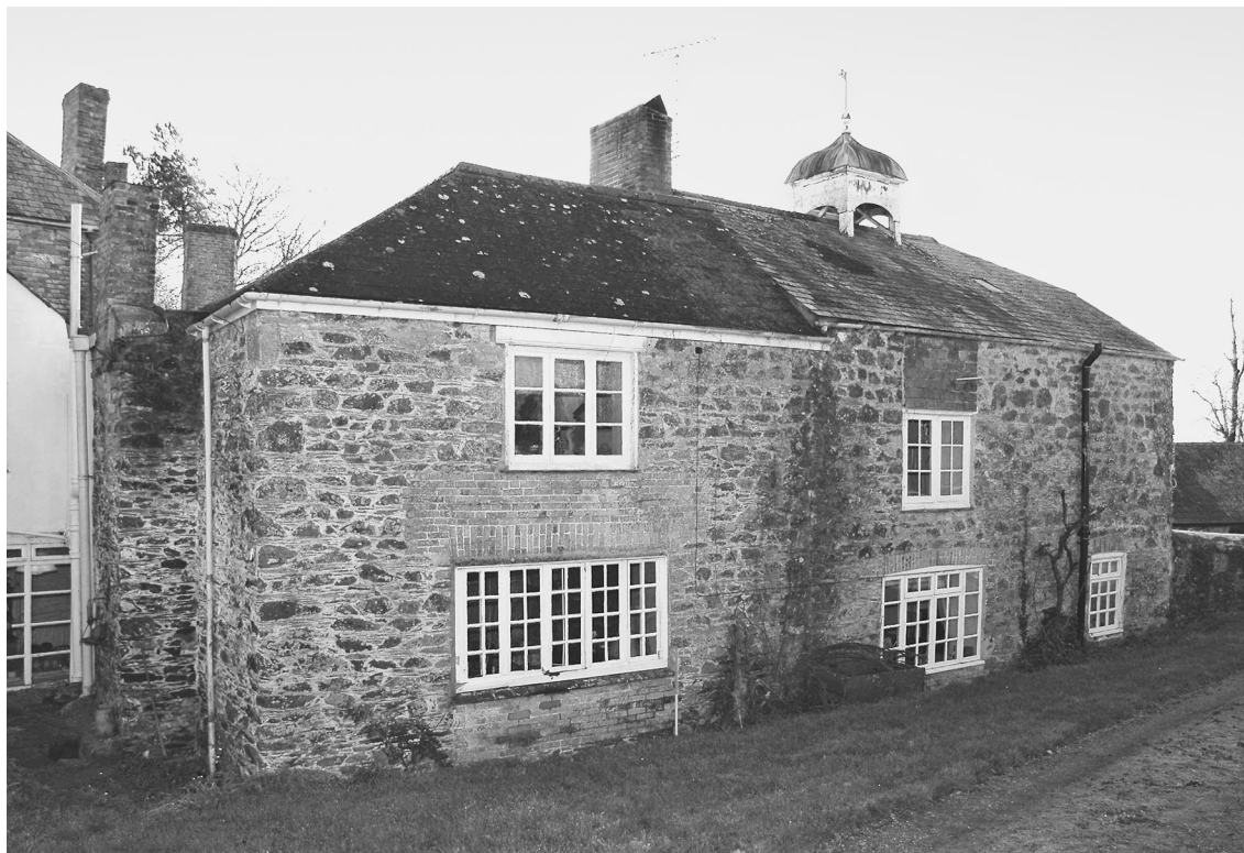
Fig 4 The north-west elevation of the sixteenth-century house (left), showing brick blocking of early window, and west range (right).
