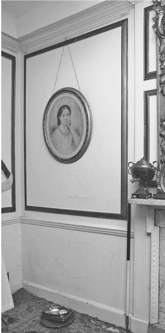
Fig 15 The east range dining room showing bolection-moulded panelling.
