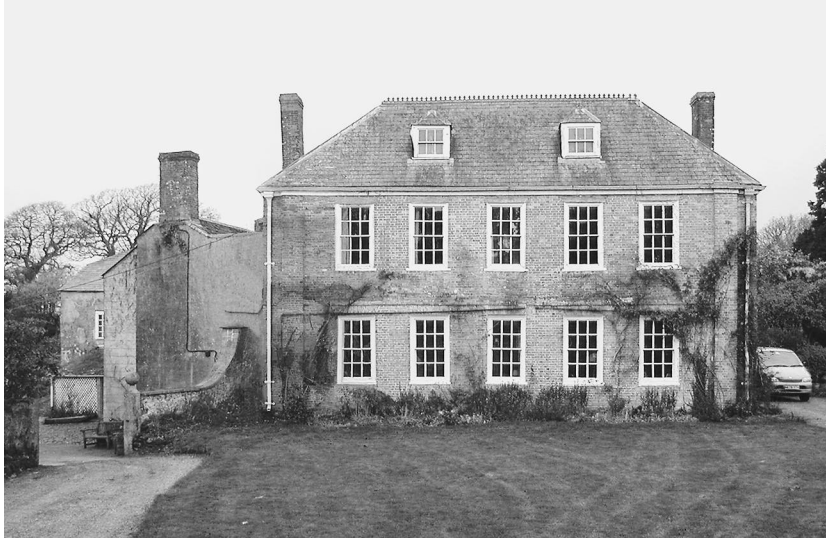
Fig 2 Hatt viewed from the south-east, with the eighteenth-century east range to the right and the gable of the older range to its left.
