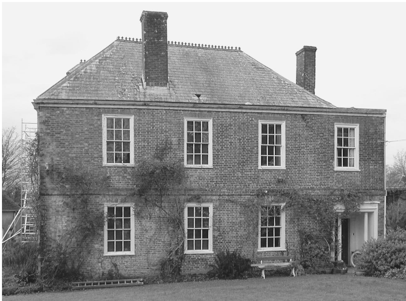
Fig 12 The early eighteenth-century east range, with later extension and porch to the right.
