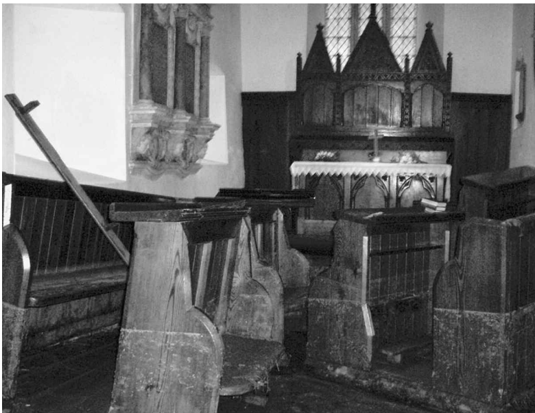
Fig 3 The interior immediately after flood damage, 17 August 2004, showing displaced pews (photograph: R Clark)
