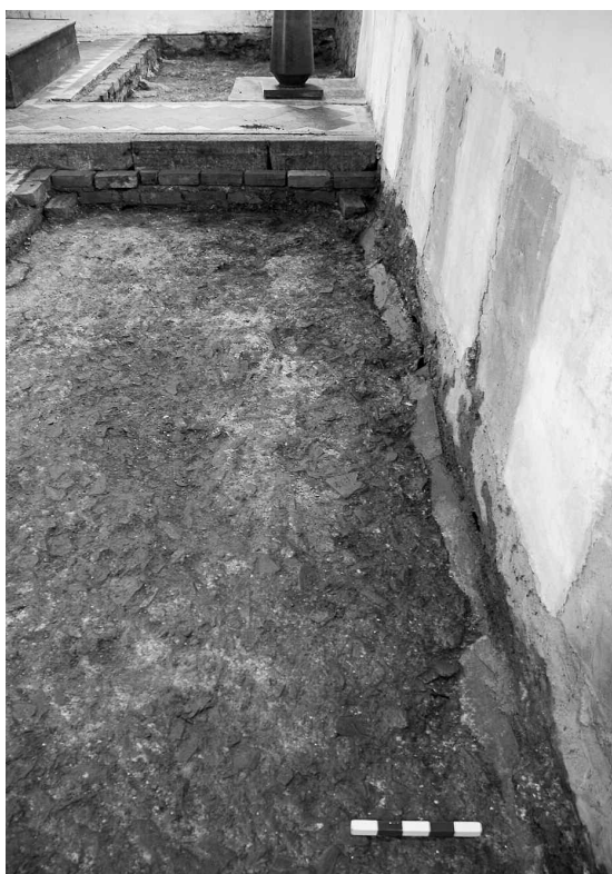
Fig 7 Drain along the internal face of the south wall (photograph: G Young)
