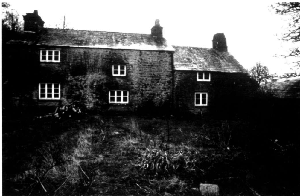
Fig 13 Stonaford; the original front (but present rear) with its 17th-century eaves line on the right, otherwise heightened (photo by Eric Berry)
