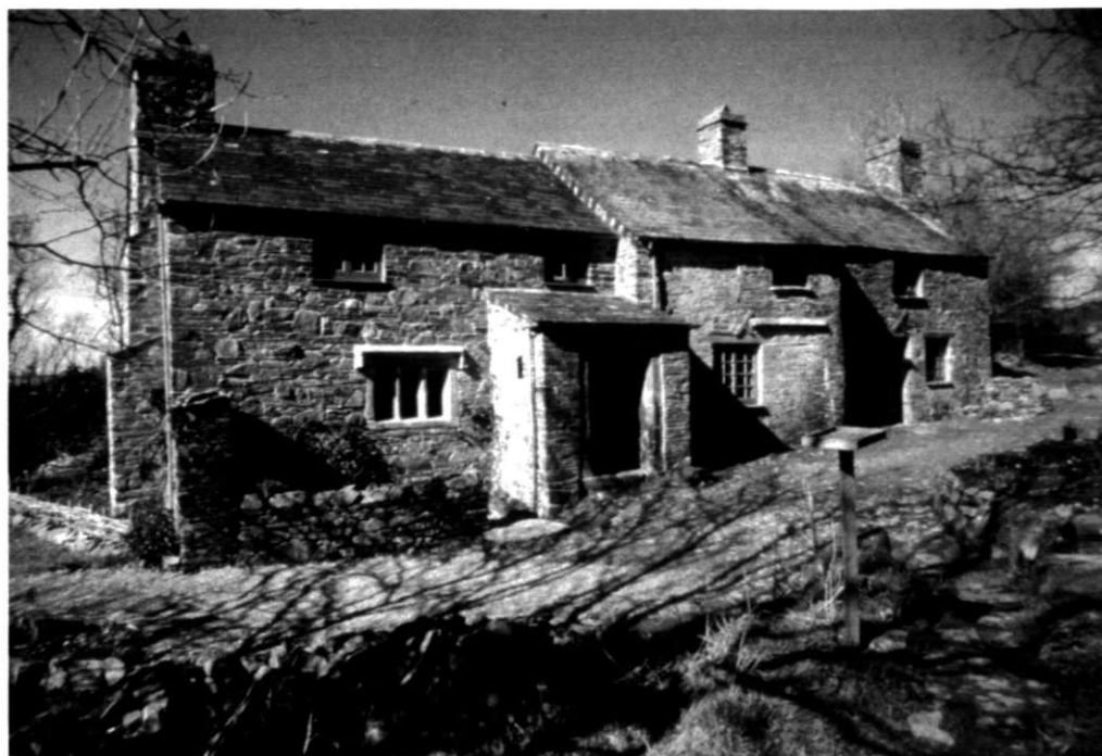
Fig 12 Halbathick after renovation and rebuilding of the lower end, the lower part of the front masonry having been numbered and reset in its former position, the porch doorway and mullioned window re-discovered on site and re-assembled (photo by Eric Berry)
