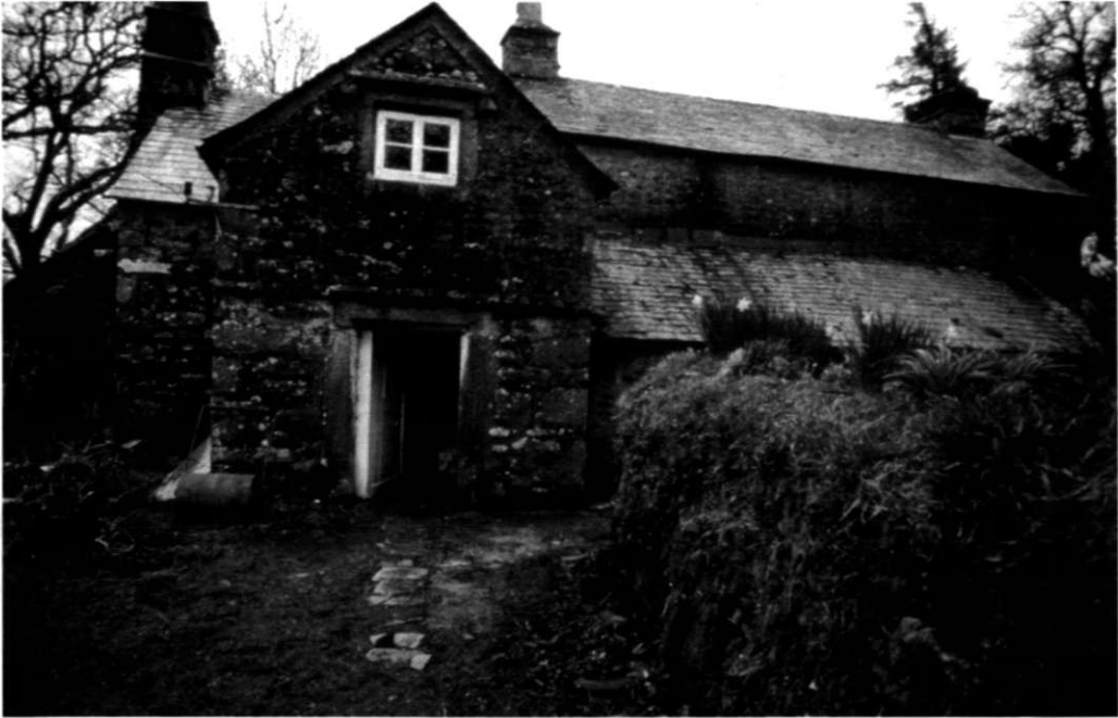
Fig 14 Stonaford: 17th-century entrance porch fronting the lower end, originally the shippon and likely to have been one roof bay longer to the left (photo by Eric Berry)
