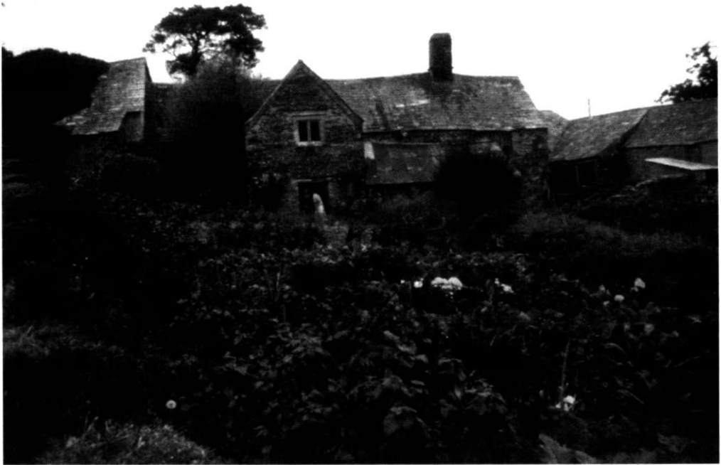
Fig 9 Cullacott; rear elevation (the original front) prior to collapse of large areas of wall. Renovation works were undertaken in 1995 and 1996 (photo by Eric Berry)
