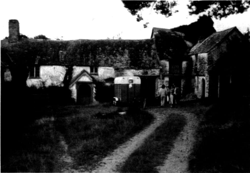
Fig 10 Cullacott; the courtyard front in the late 1980s. The lower end (the original shippon) is left of the porch, the open hall right of the porch, and the parlour at the far right with wing in front (photo by Eric Berry)
