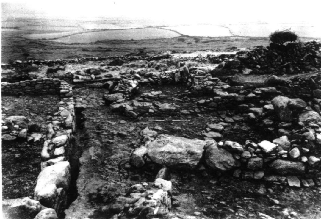
Fig 10 Old Lanyon. The Cot (House 2) looking north-west.
