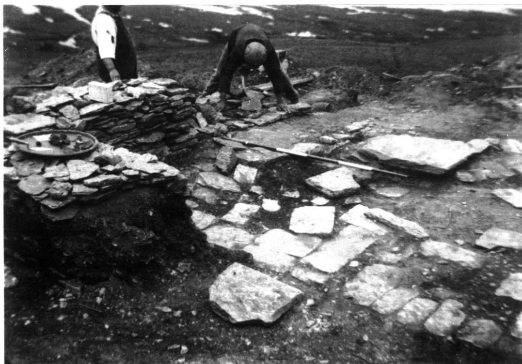
Fig 10 Lammana chapel 1936. The chancel, with surviving northeast corner of wall, paving, and end of altar block, on which ranging rod (scale of feet) has been placed. Note that here as elsewhere slates have been piled on remaining walls, and that a workman is placing stones to mark the inner line of the east wall behind the altar
