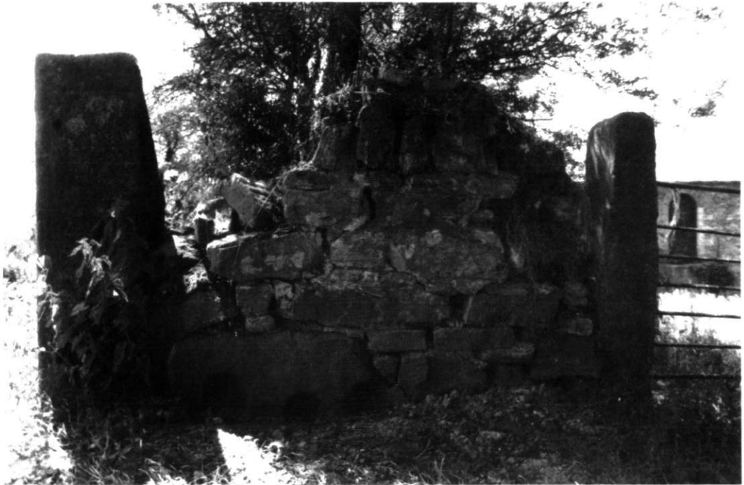
Fig 9 Mortar stone from Trevithick
