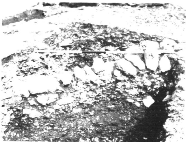
IX MIDDLE RAMPART ENTRANCE, EAST SIDE: LIGHT REVETMENT WALL
