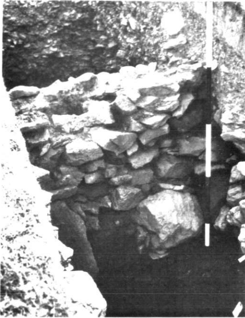
V MIDDLE RAMPART; STOUT REVETMENT WALL AT TAIL OF BANK (NOTE SANDSTONE BLOCK WITH IMPRESSION OF MISSING STONE)
