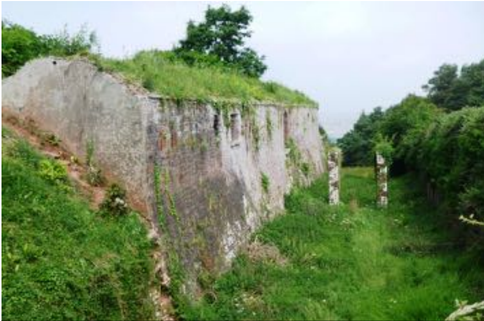
Redoubt 5: view down eastern moat
