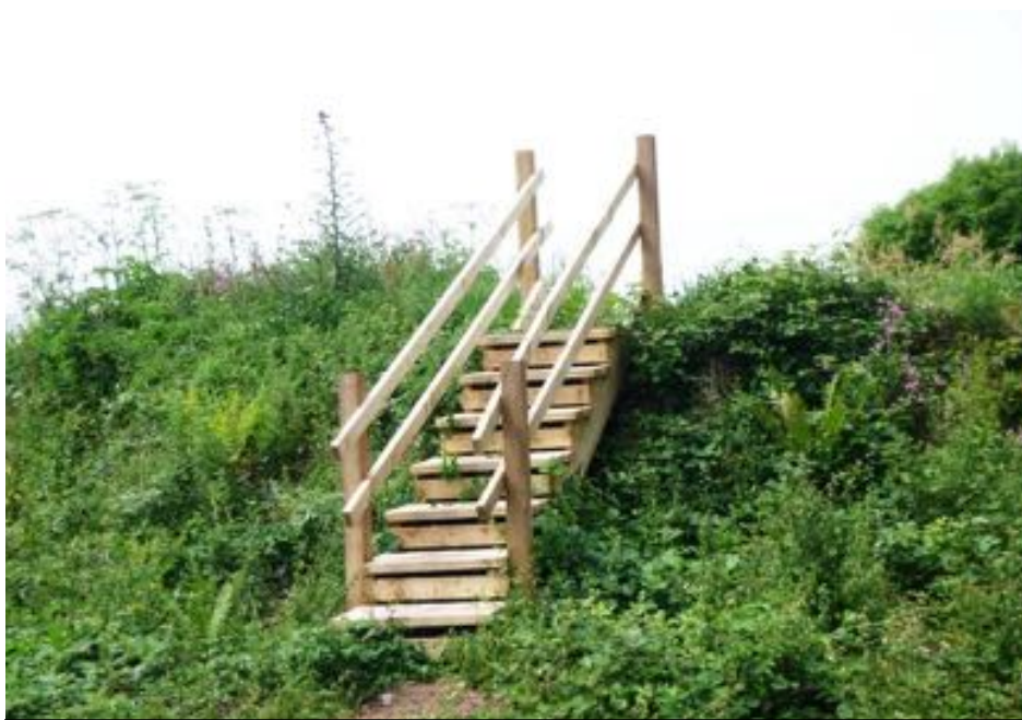
Redoubt 3 – View of access steps
