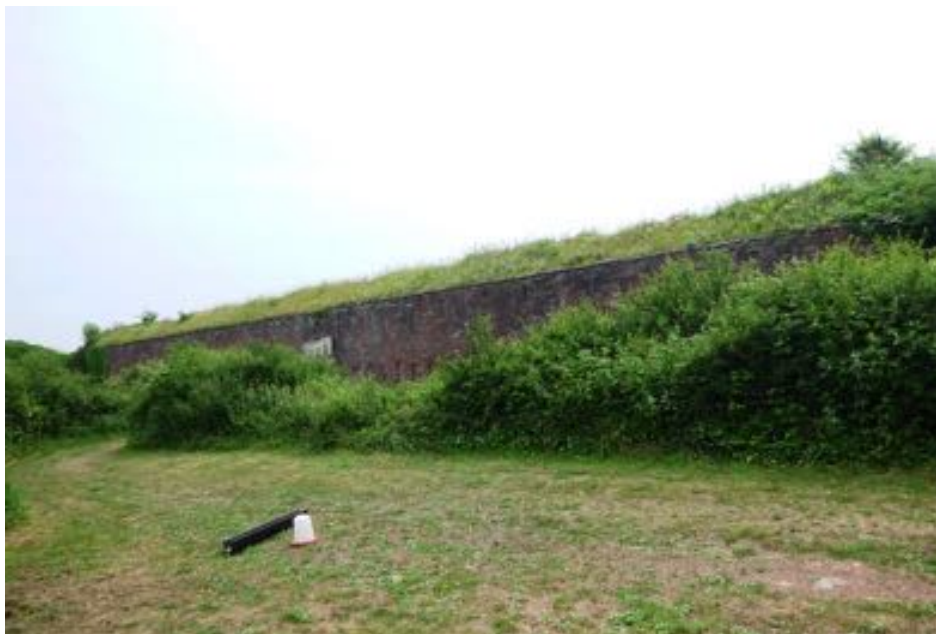
Grenville Battery – front view
