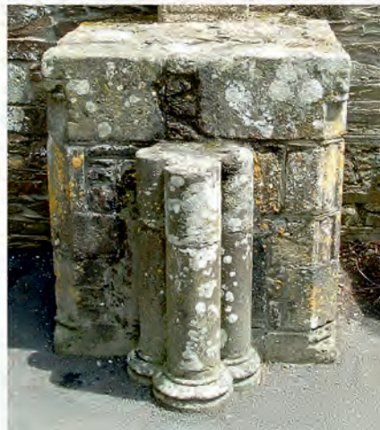
Fig 3 Profiles of engaged shafts and responds, with view of the south-western respond of the Lady Chapel (Respond 1), rebuilt beside St Thomas church. (Drawings and photograph: J Allan.)
