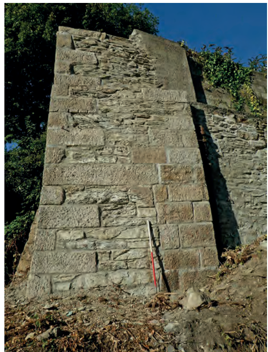
Prospect Place, Falmouth. An impressive section of walling and buttress, probably dating to the mid-eighteenth century, reprinted after being revealed by site clearance work. (Photograph: © Cornwall Archaeological Unit.)
