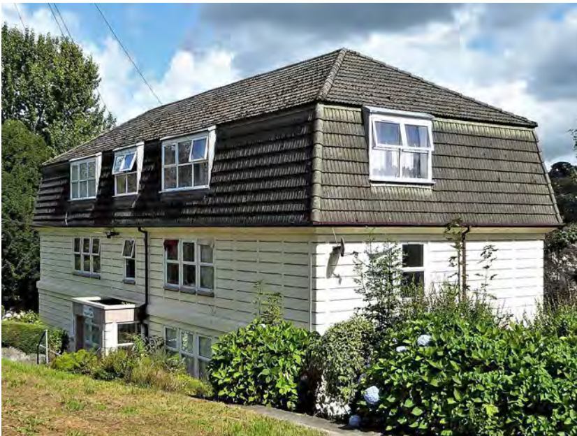
Cornish Unit flats at 1–11 Polgrean Place, St Blazey. (Photograph: Graeme Kirkham.)
