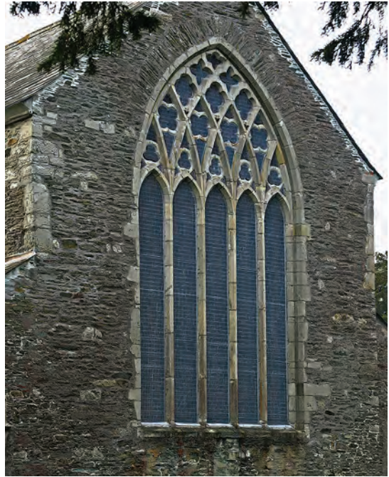
Fig 30 Church of St Bartholomew, Lostwithiel. Late thirteenth-century east window, constructed from Pentewan stone like many of the dressed fragments found at Restormel Castle. (Photograph: Eric Berry.)
