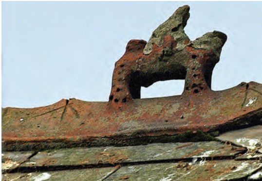
Fig 22 ‘Horse-and-rider’ crested ridge tile on the taller roof of the Jolly Sailor public house in West Looe, one of three horse-and-rider examples that survive in Looe; the only other known examples are in museum collections. (Photograph: Eric Berry.)
