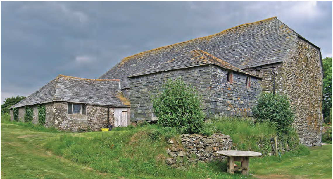
Fig 27 Bokelly Barn, St Kew, horse-engine house and granary; rag slate throughout plus rag slate-hanging on granary. (Photograph: Eric Berry.)
